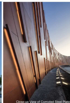
Close-up View of Corroded Steel Plate
