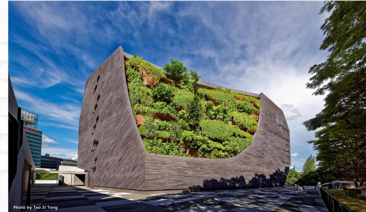
Green wall facade at LKC Natural History Museum, Singapore depicting the native cliff landscapes along the coasts Image courtesy Tierra Design
